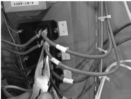
Using a Philips screw driver (Cross), unscrew the red (-Negative) & Yellow (+ Positive) wires from the oval ceramic thermo couple block.
